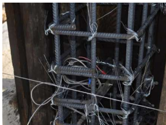
Figure 5: Insertion of a thermocouple
