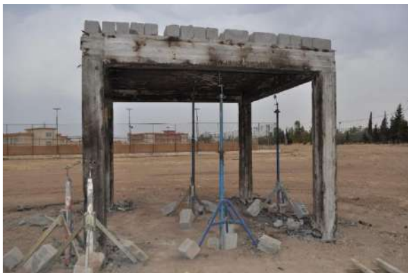
Figure 13: Location of installed dial gauges
