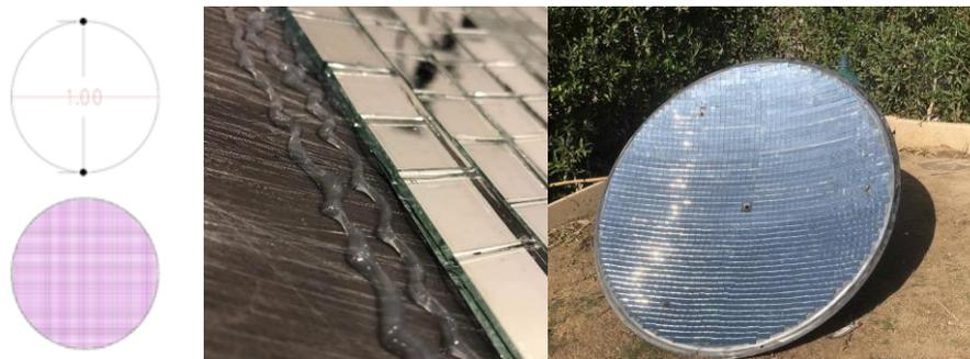
Figure 2: Design and install mirrors on the dish surface
