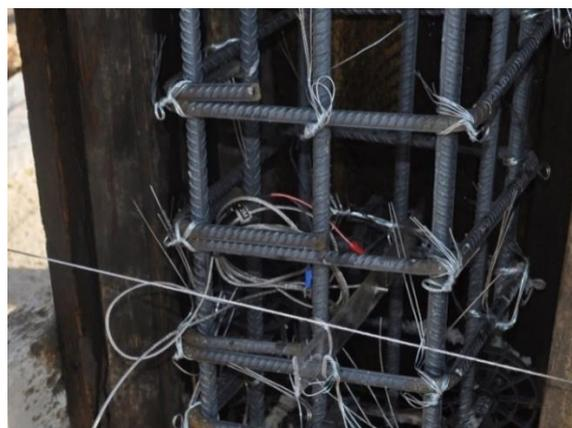
Figure 5: Insertion of a thermocouple
