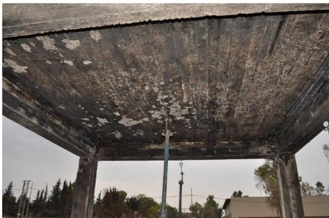
**Figure 16:** Spalling and change color occurred in slab
