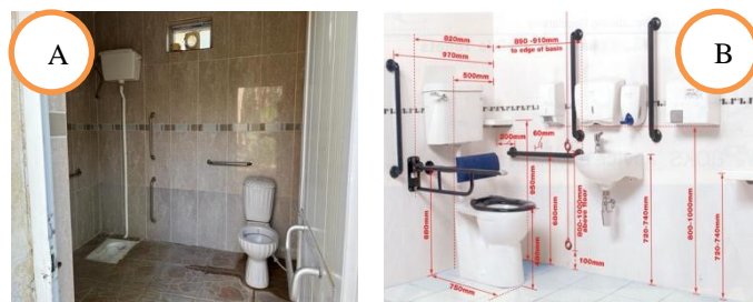
Figure 7: Toilet: A) Only exiting ones (Source: Author). B) Proposal for future (Source: Grab Rails, 2023).
