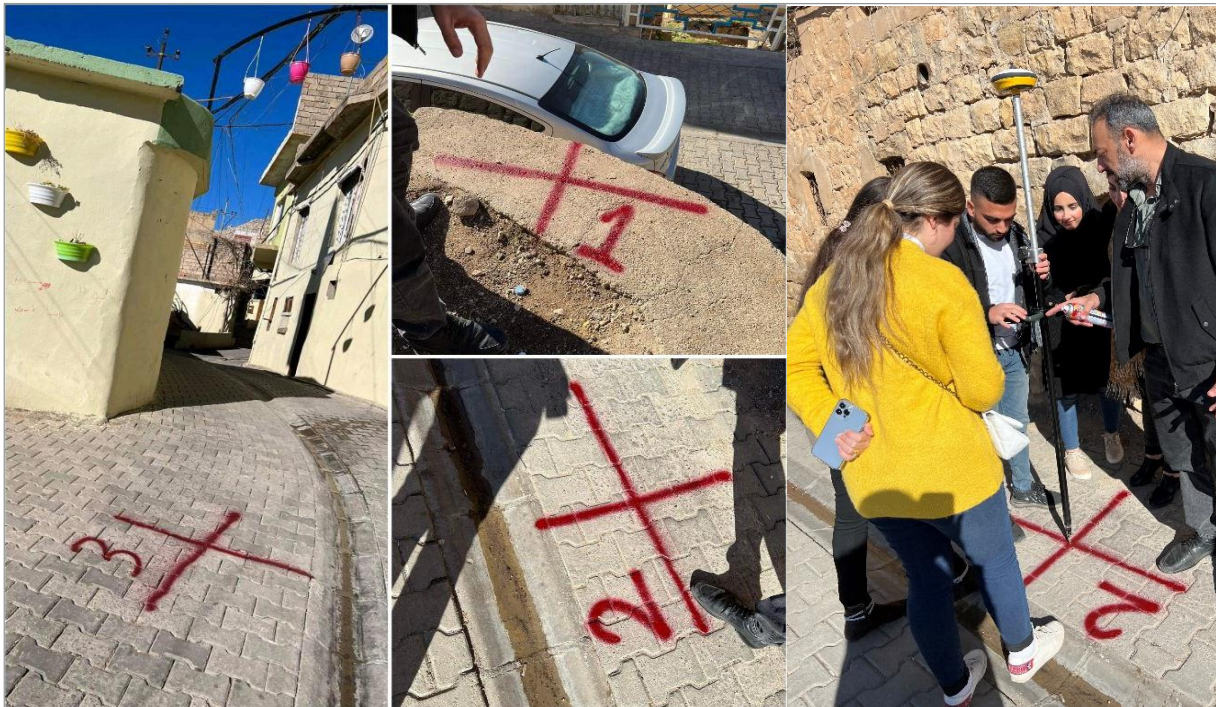
Figure 06: GCPs Marking and surveying using instrument eSurvey E200 GNSS
